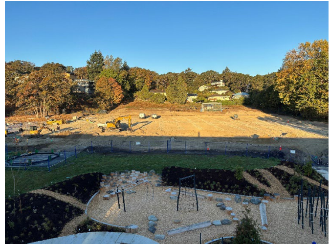
Image 2 – Playground install / Field Progress
