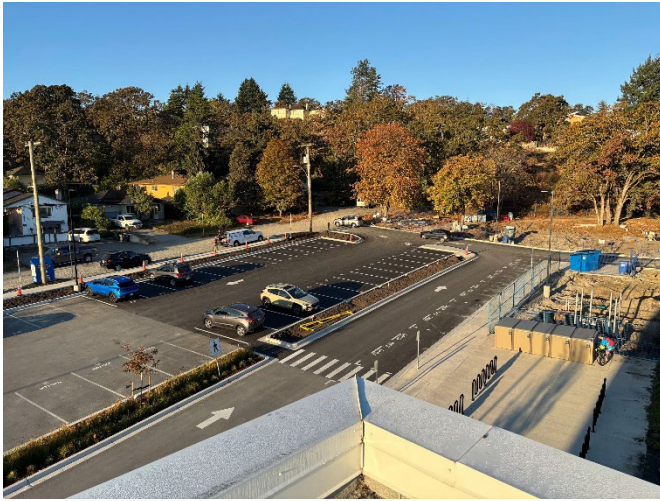
Image 1 – Parking lot Phase 2 completion
