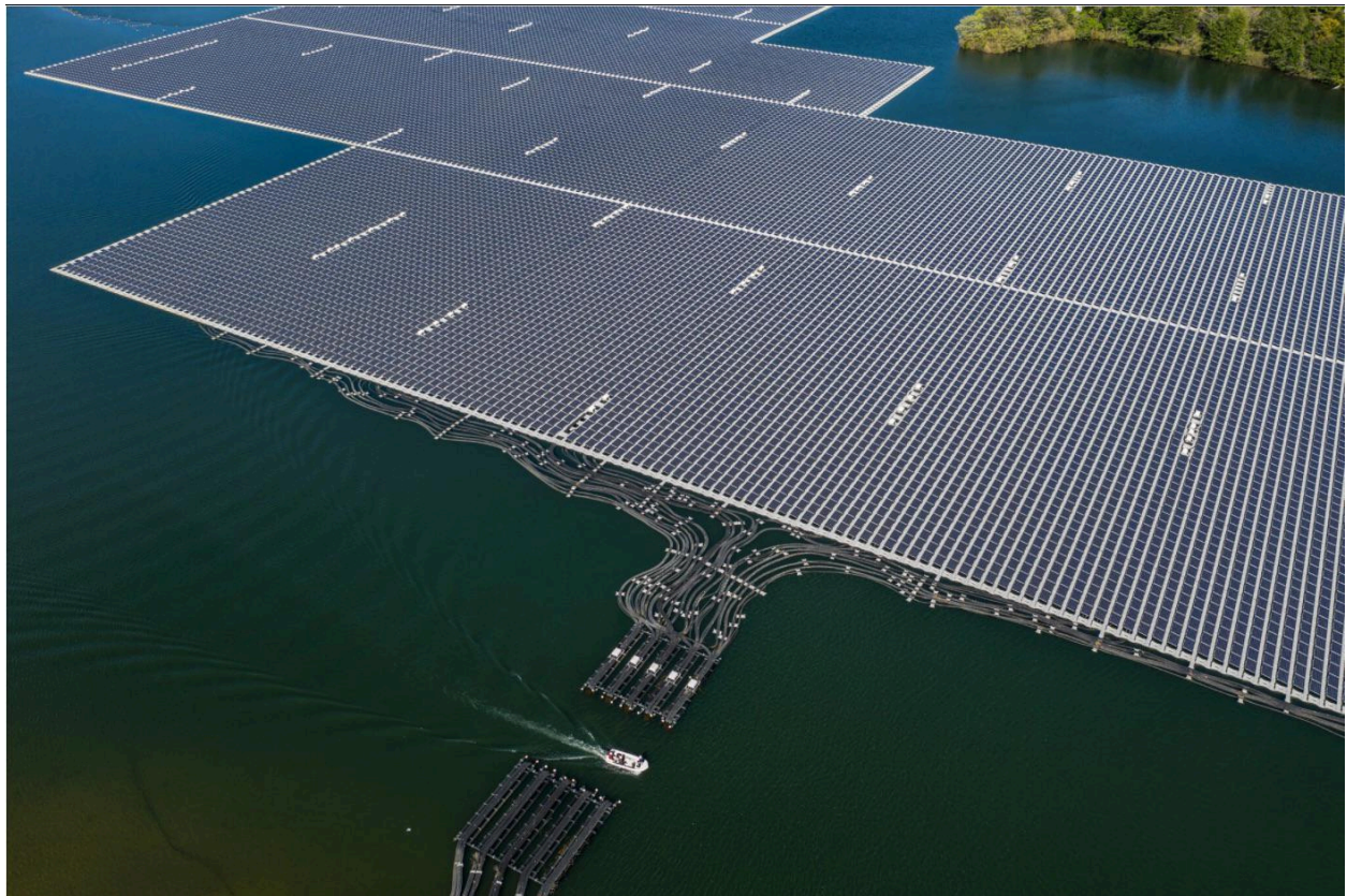
Floating solar panel farm in Japan in reservoir behind hydro-electric dam
