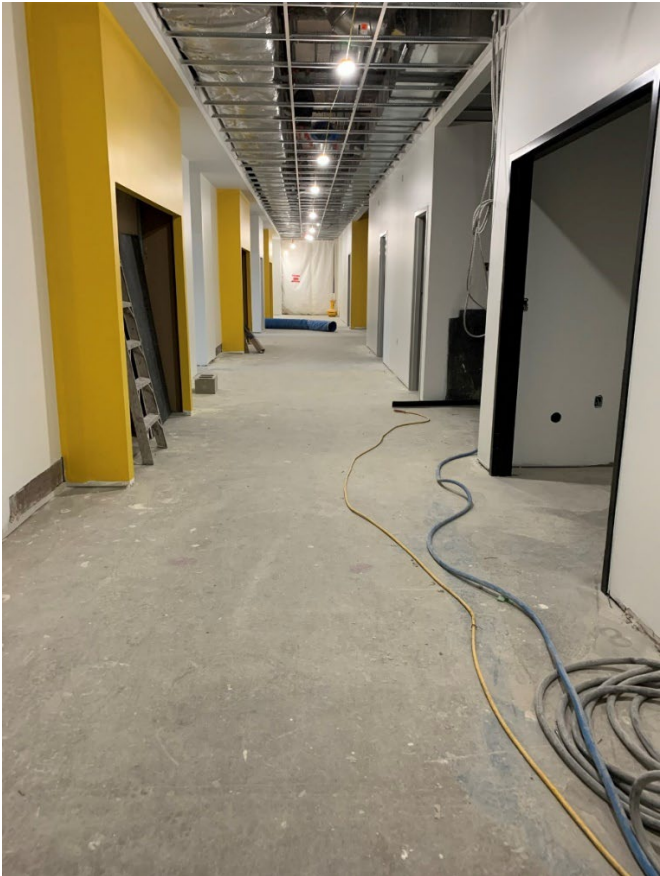
East Wing Hallway Finished Drywall and Frames
