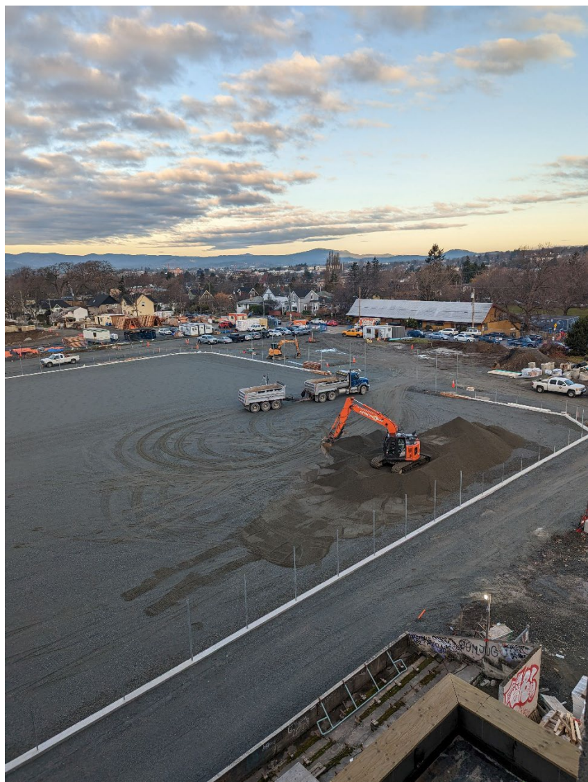
Delivery Top Layer of Gravel for the Turf Field
