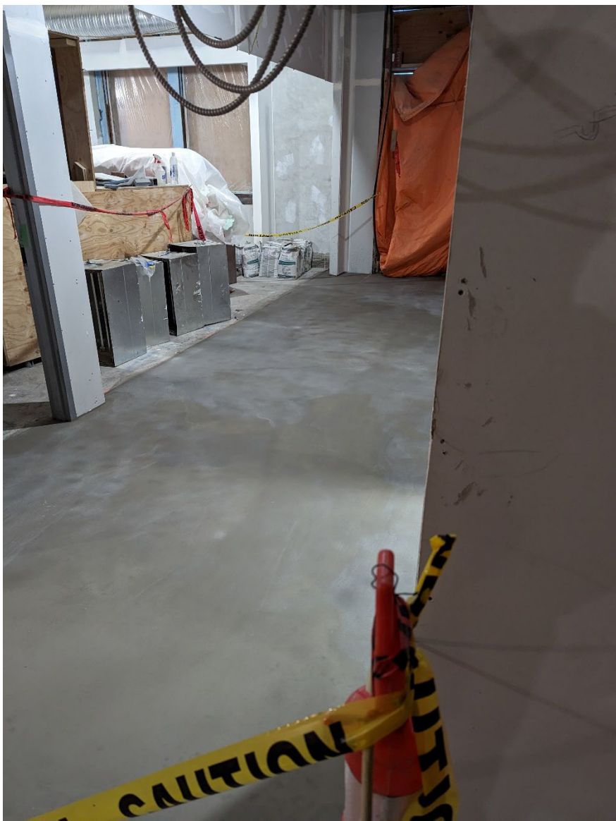
Floor Leveling on Level 1
