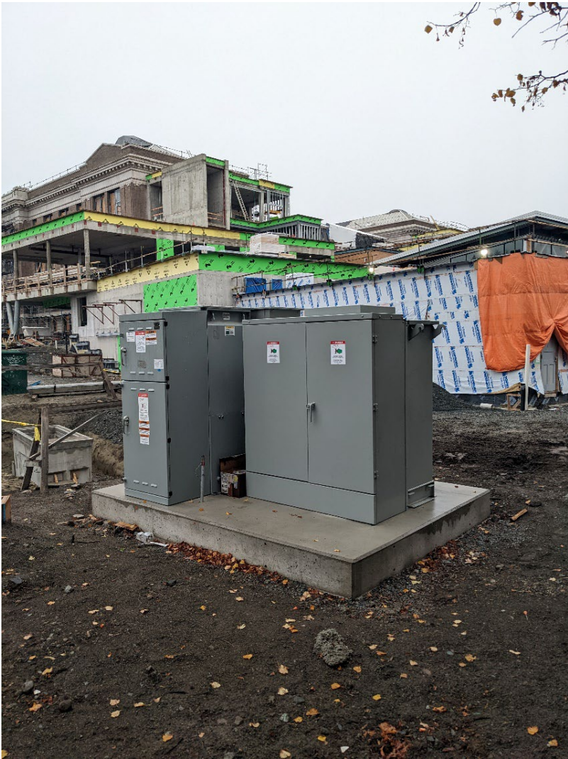
New BC Hydro Kiosk Installed
