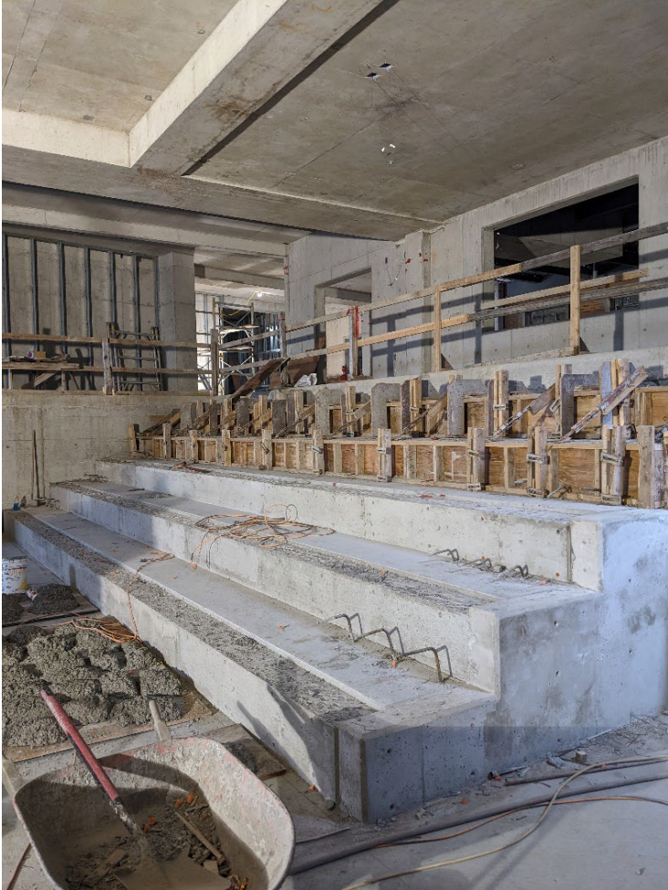
Multi-Purpose Room Bleacher Installation
