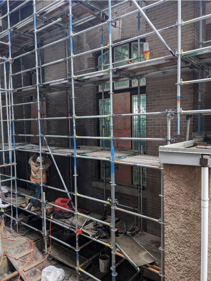
Exterior Brick and Window Refurbishment in Progress in East Lightwell
