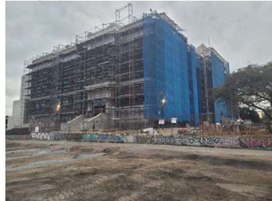
Scaffolding setup on south face for exterior envelope work
