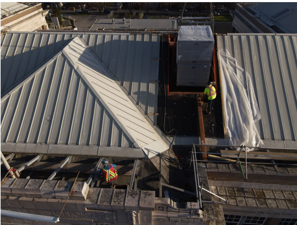
Air Handling Unit – Drop through the Roof
