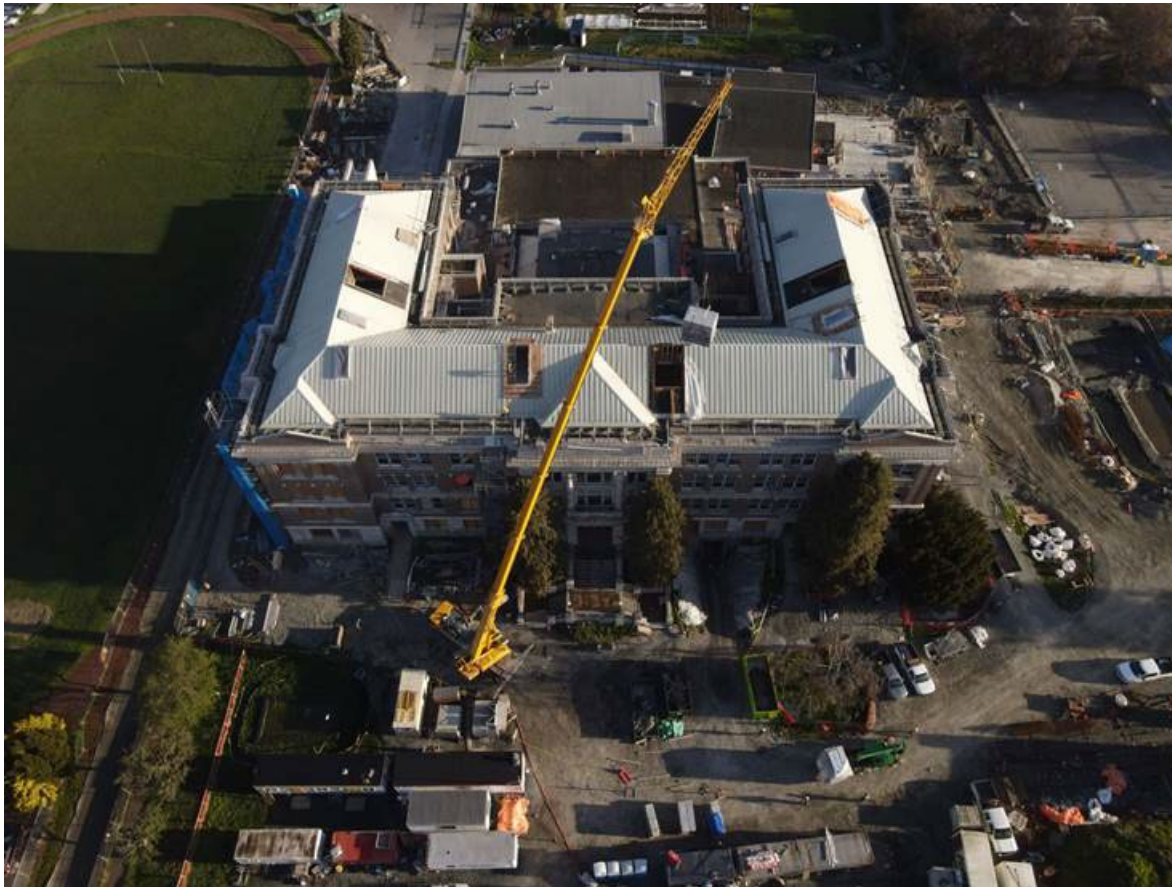
Craning used to place the heating units
