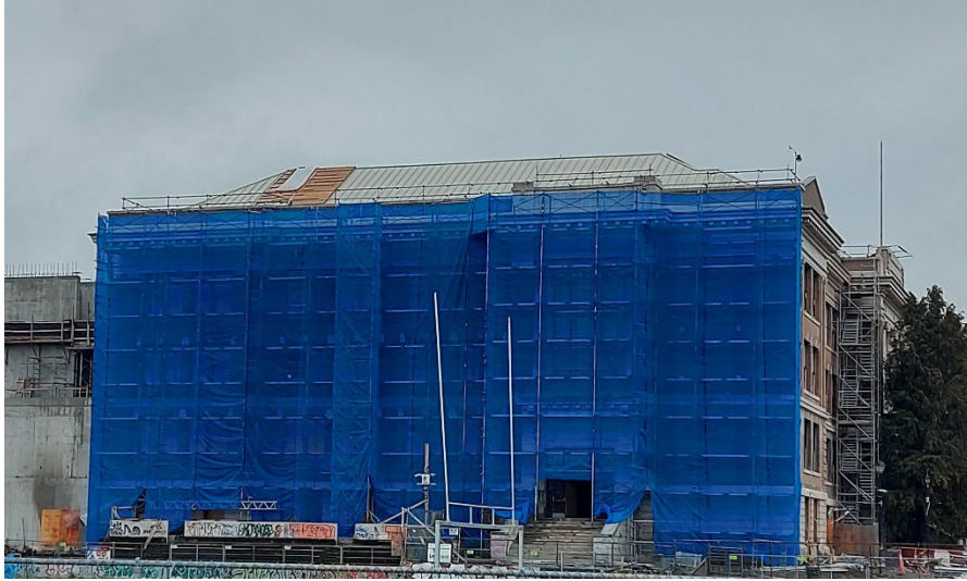
Scaffolding on West side for heritage window replacement
