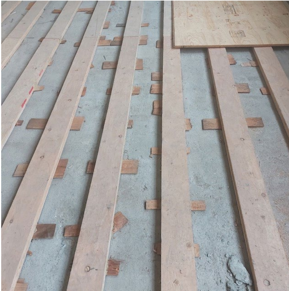
Rebuilding Classroom Floor Substructure
