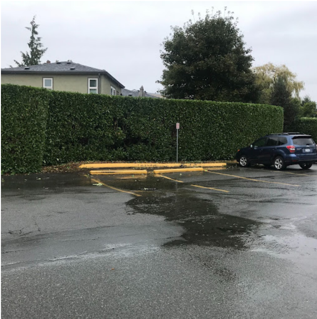
Parking lot drain overwhelmed by flooding water likely contaminated from parked vehicles. Drain leads directly into Bowker Creek.
