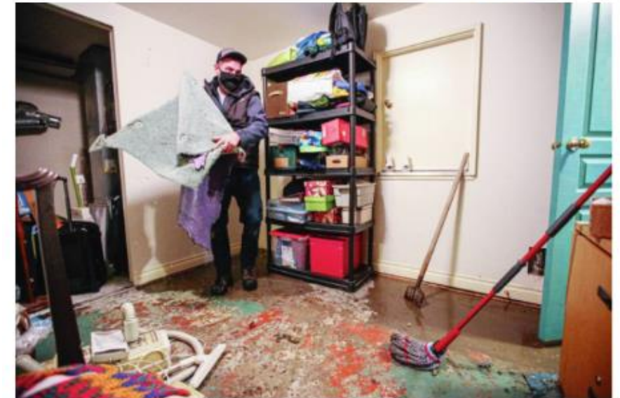
Jason Morrow with Downs Construction removes soaking wet carpet liners from a home on Pacific Street in Oak Bay after flooding along Bowker Creek. ADRIAN LAM, TIMES COLONIST
