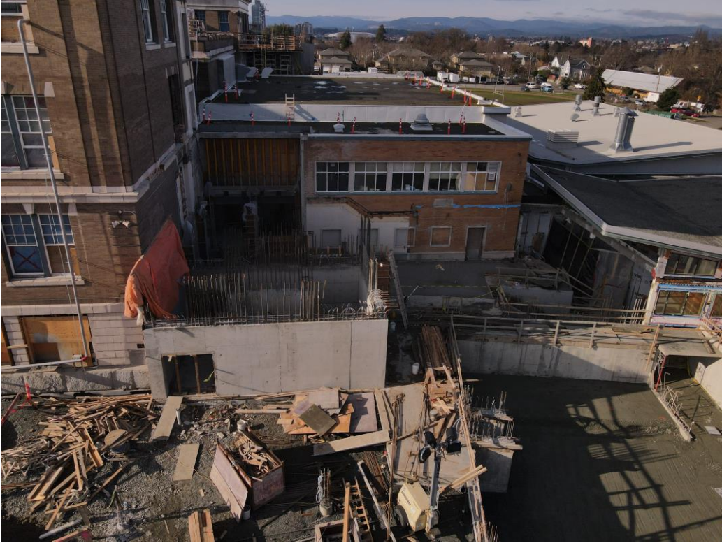
February 2022 – Drone View – East Stair Tower
