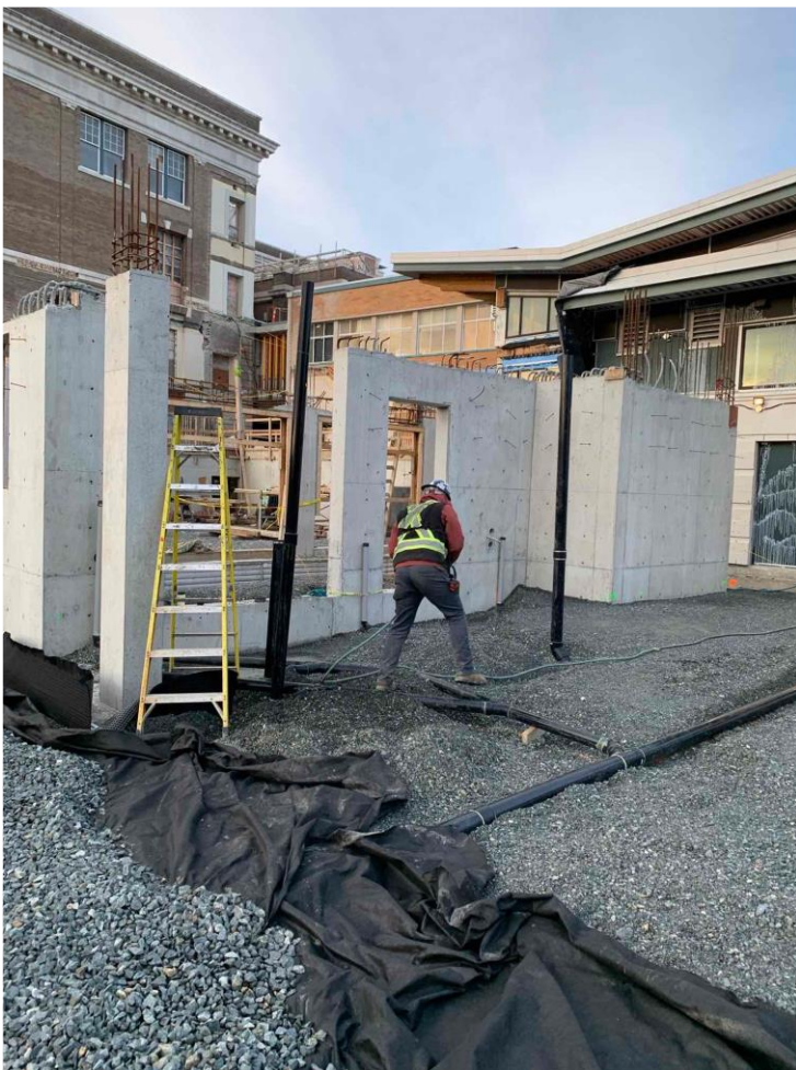
December 2021 – NLC Building – Slab on Grade Underground Piping Installation
