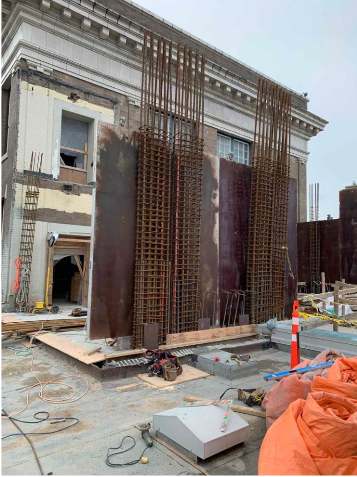
December 2021 – Stair #1 – Level 3 Concrete Walls Being Formed
