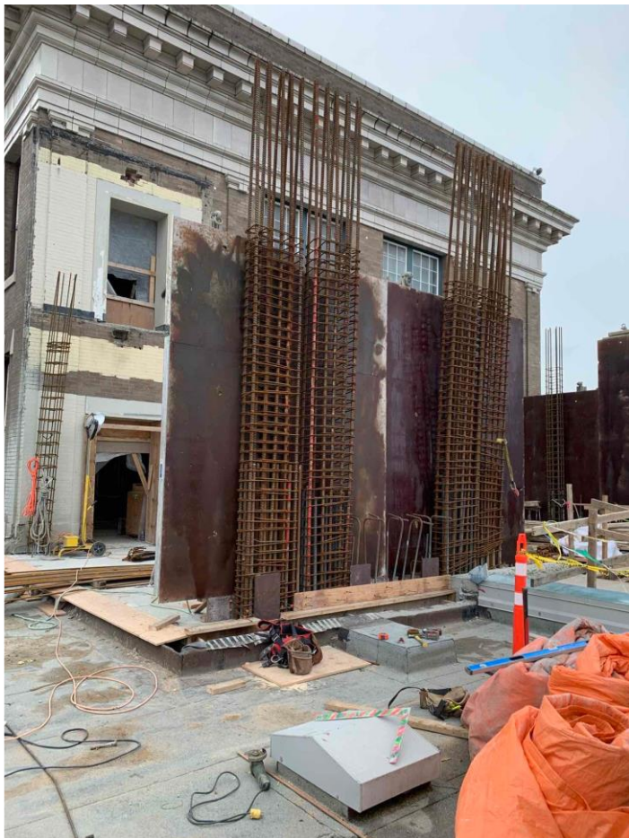
December 2021 – Stair #1 – Level 3 Concrete Walls Being Formed
