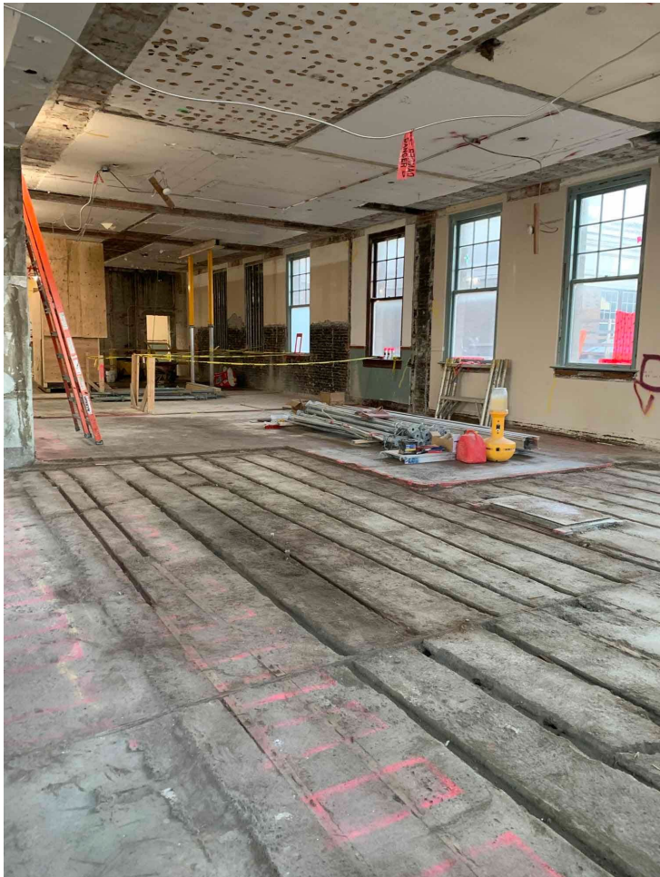
November 2021 – Wood Flooring Removed Leaving Concrete Floor with Sleeper Trenches
