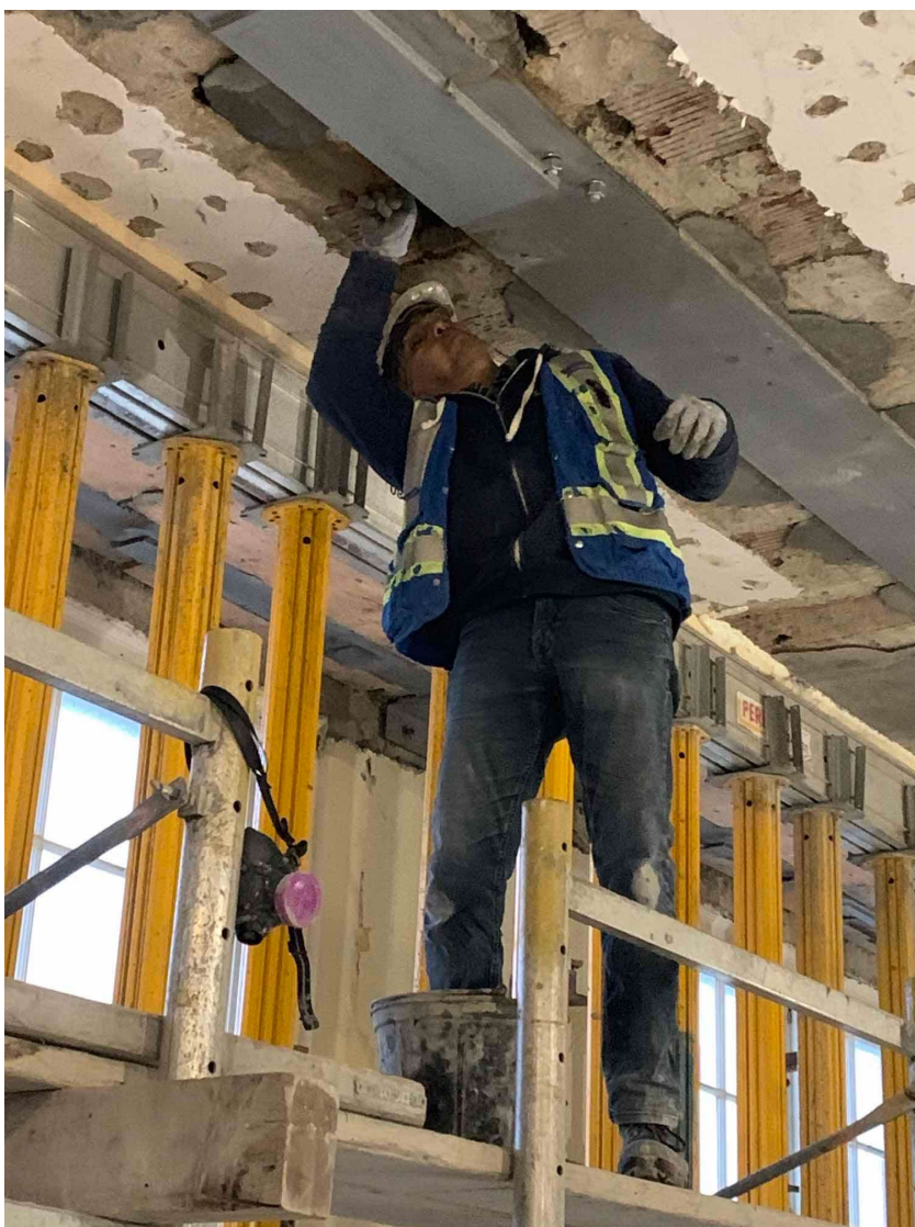
November 2021 – Concrete Patch for Drag Strut
