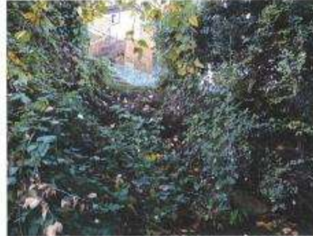
South-west corner of the Kachan property. Much of this corner has eroded away in recent years.
