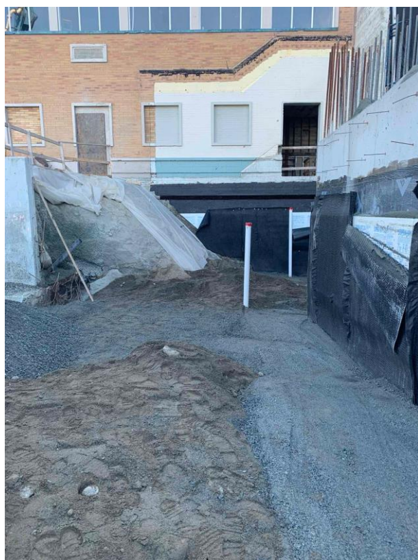
August 2021 – Backfill and Waterproofing at NW Stairs
