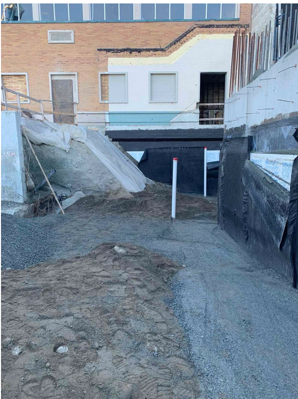
August 2021 – Backfill and Waterproofing at NW Stairs
