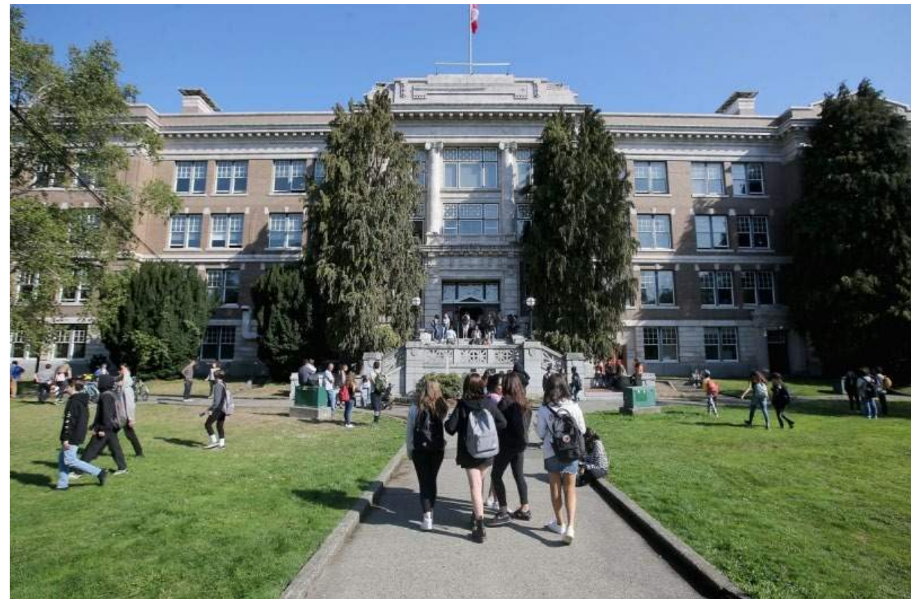
Original Main - Grant Street Entrance
