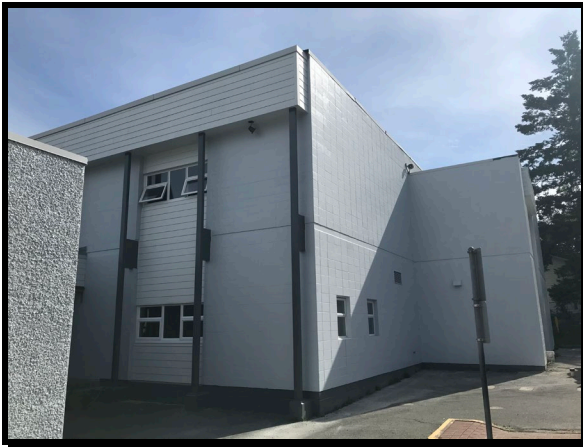
New Exterior Paint
