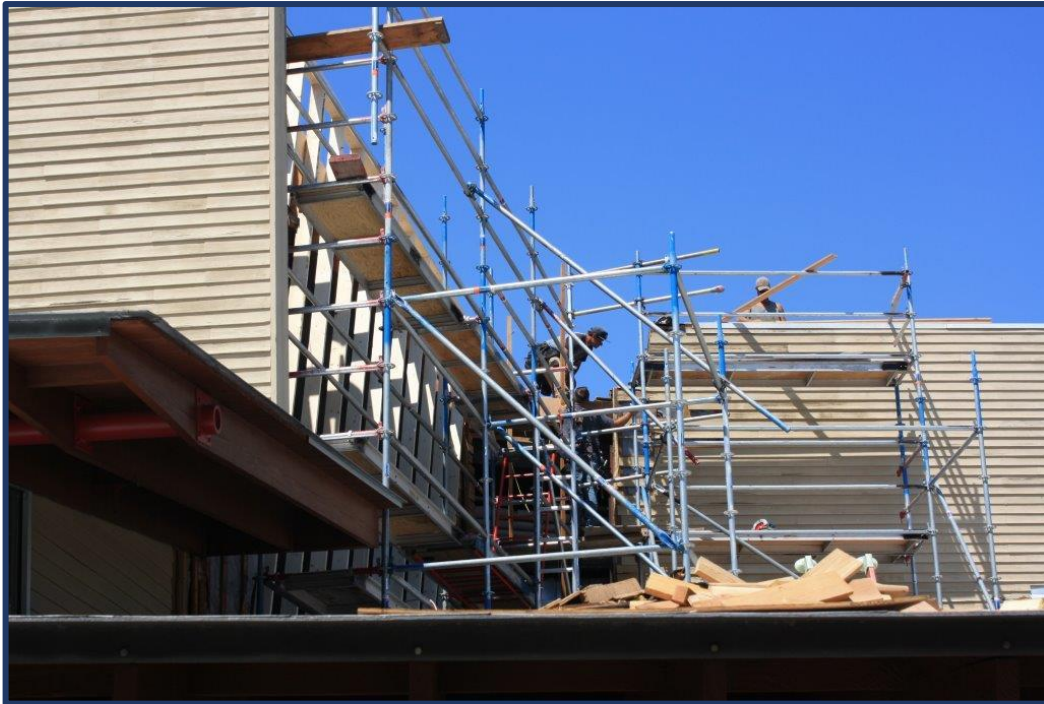
Removing all burned Roof Joists and Exterior Wall Siding
