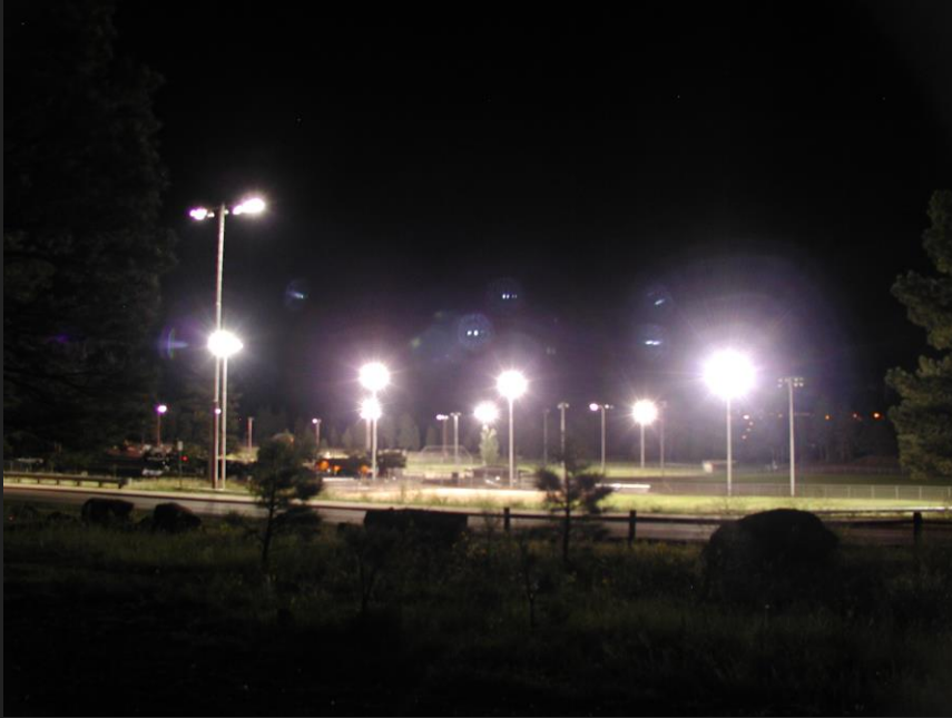
Old unshielded HPS sports field lighting showing light wash in the foreground
