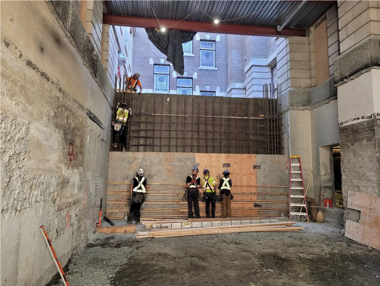
June 2021 – Lower level of new concrete shear wall at Interior Atrium/Roper Gym
