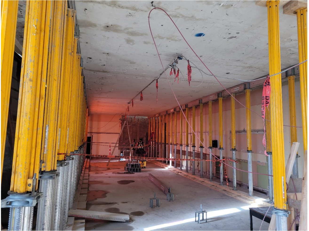
June 2021 – Lines of re-shoring at lower level
