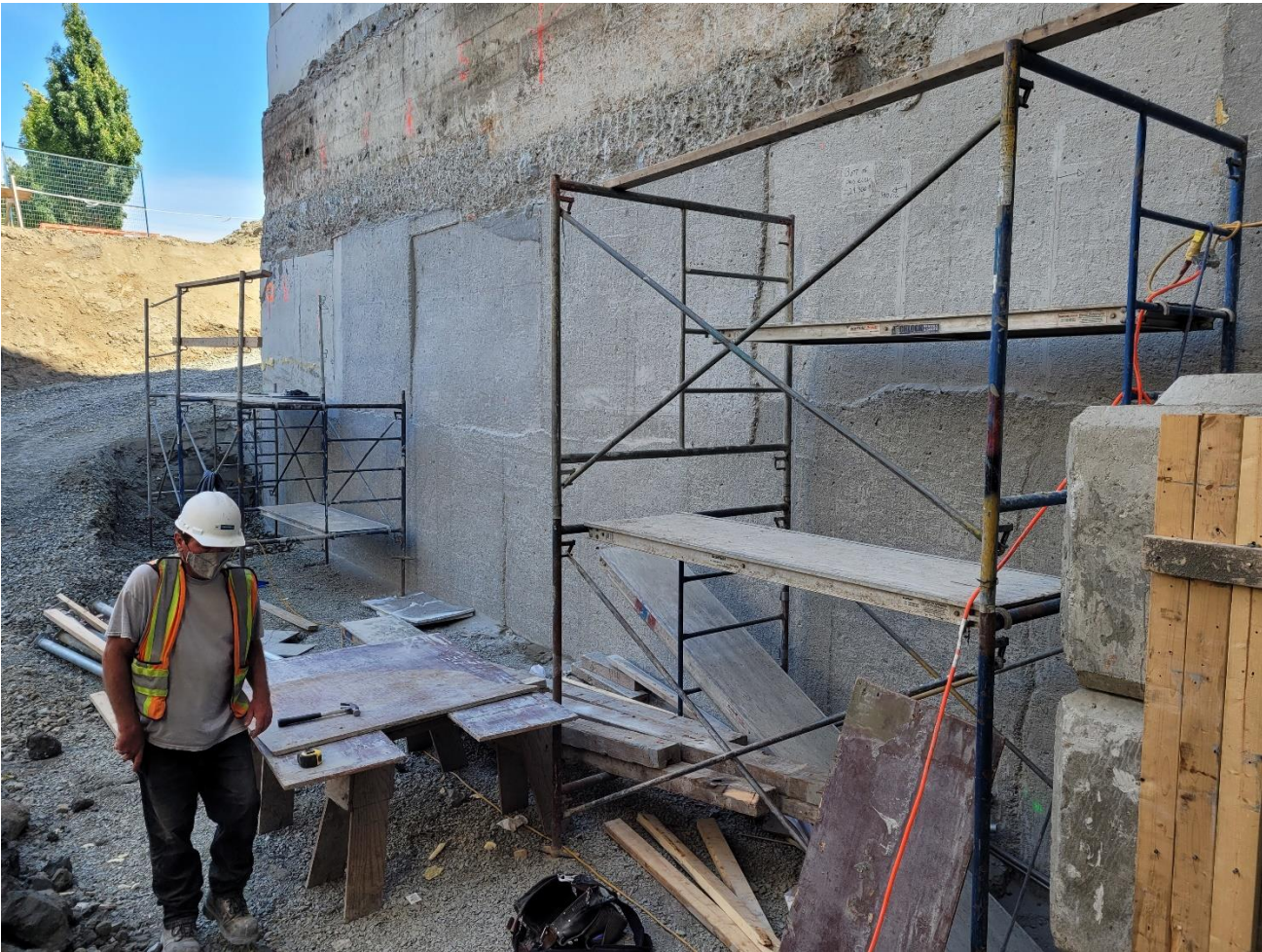
June 2021 – Concrete underpinning of old footings at NE corner of school. The rough concrete seen at about the top of the scaffolding is the old footing.
