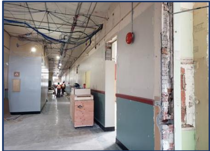
Typical sample of corridors having been stripped for abatement
