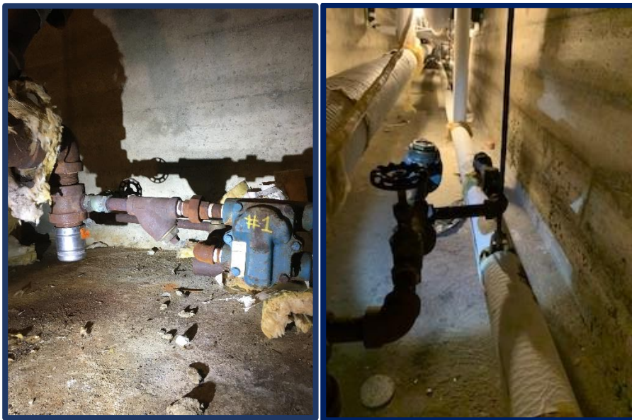
Steam Piping and Steam Traps Under SJ Willis
