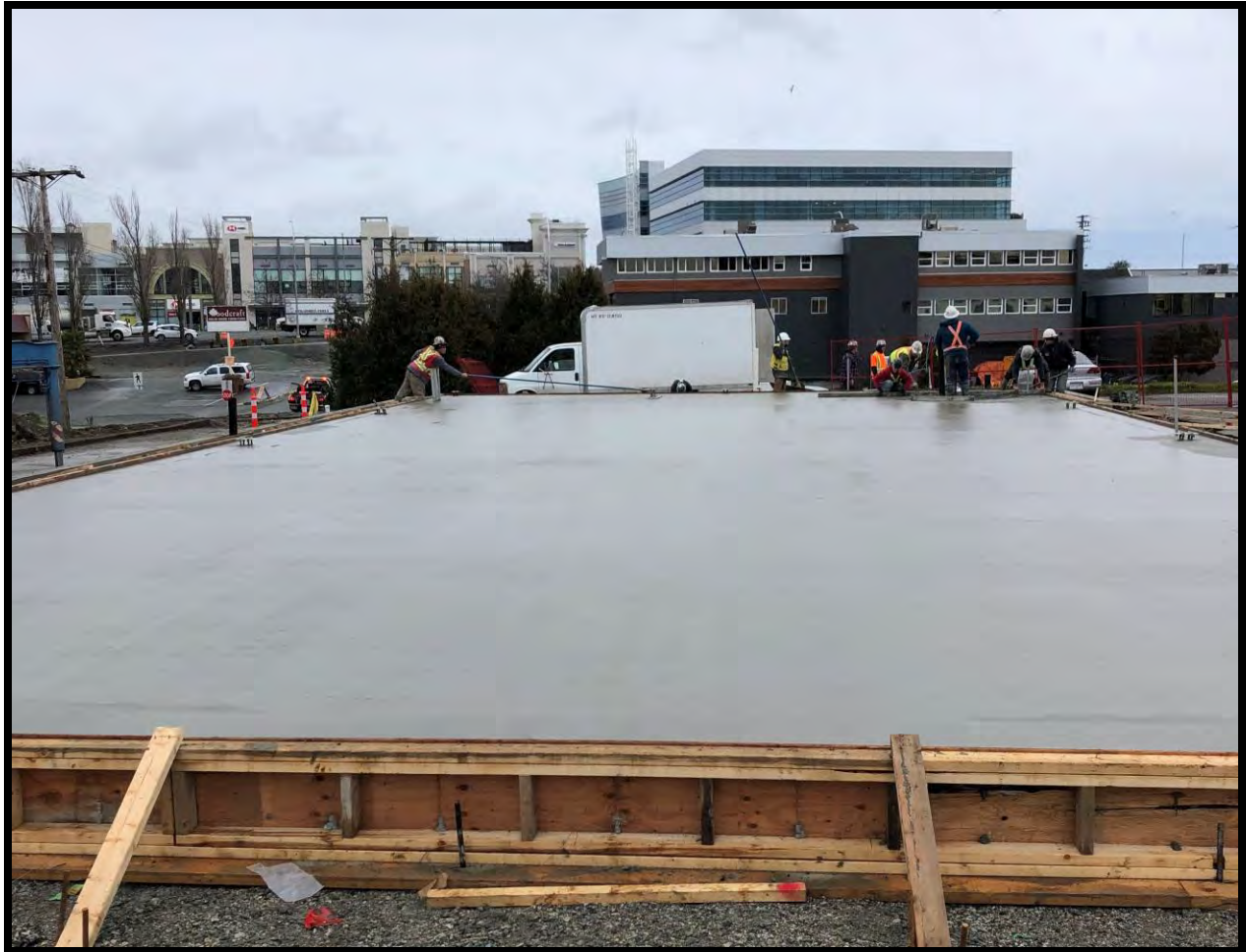
Completed concrete slab (floor) at Tolmie Trades Training Centre
