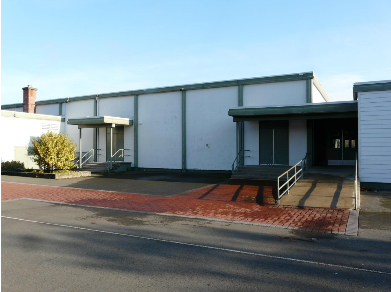
Figure 2.1: West Elevation Block #44-2 Gymnasium Uplands Elementary School
