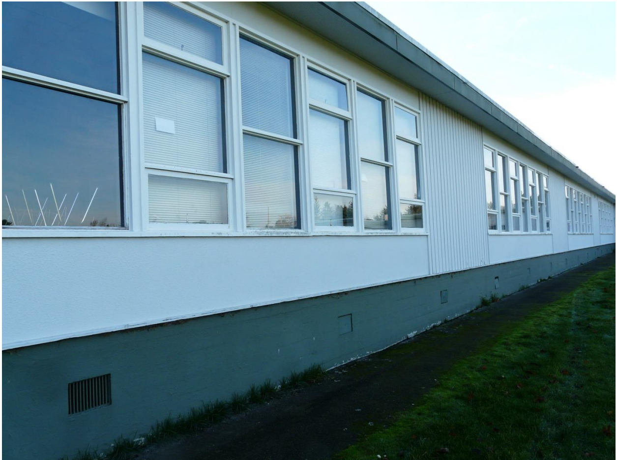
Figure 2.1: North Elevation Block #44-1 Classrooms Uplands Elementary School
