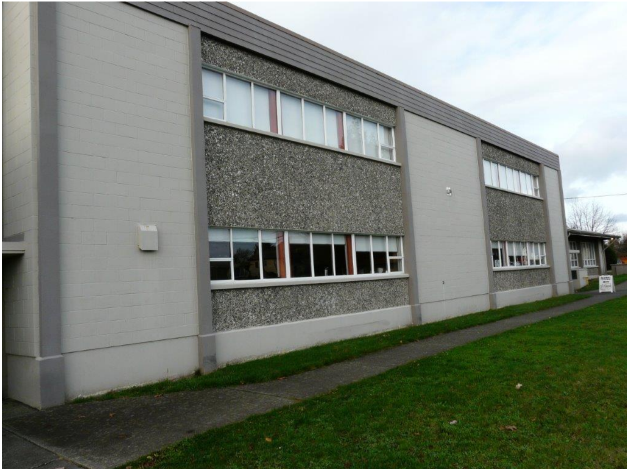
Figure 2.1: East Elevation Block #60-1 Central Classrooms Richmond Elementary School
